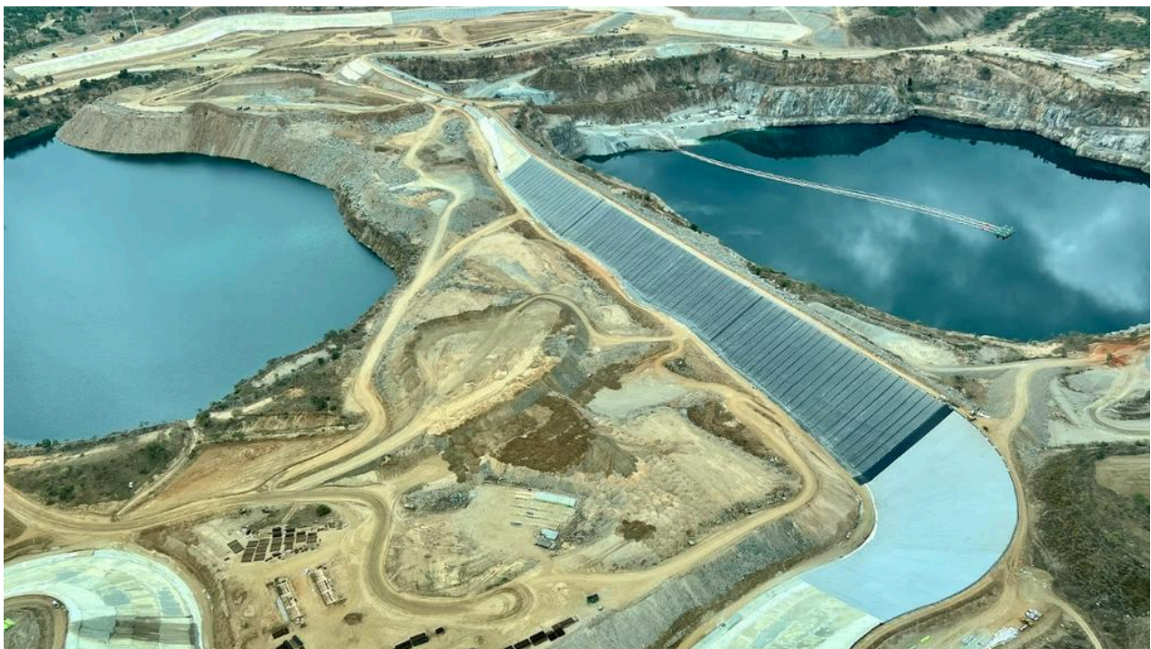
Genex Power’s 250MW Kidston pumped hydro project on the site of the disused Kidston gold mine, northwest of Townsville. An inquiry has heard efficiently connecting such projects to the grid is a better option than nuclear. Picture: Supplied
